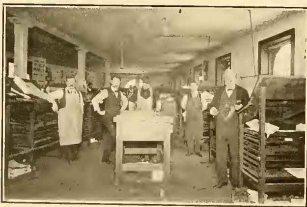
View of Job Department
