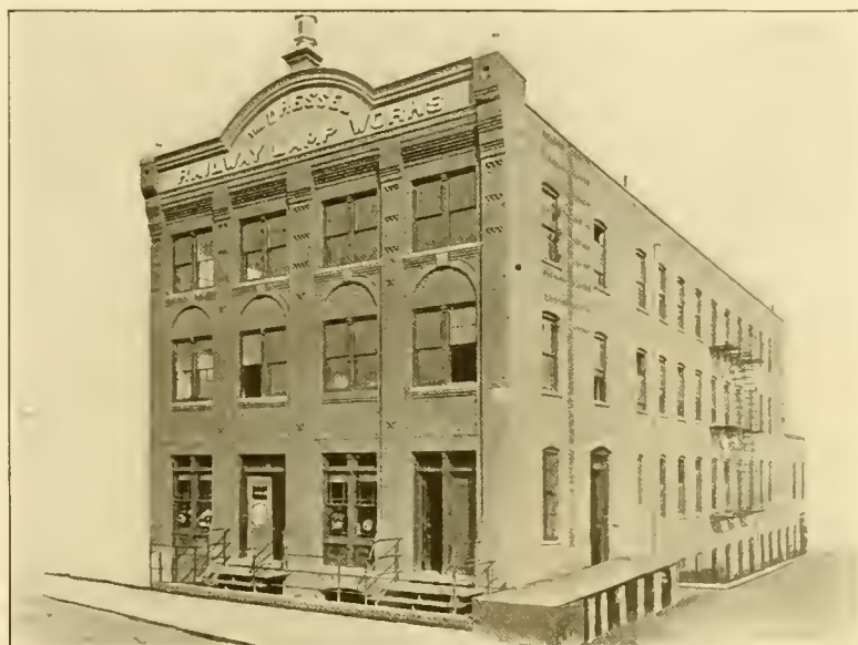
Dressel Railway Lamp Works
