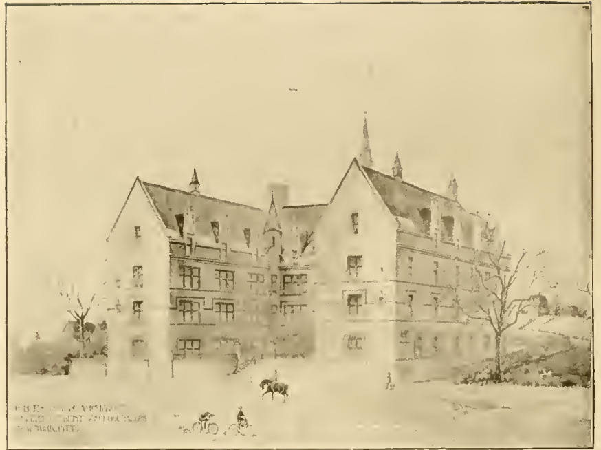
Public School No. 33, Jerome and Walton Avenues
