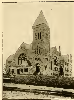
Old M. E. Church, Williamsbridge
