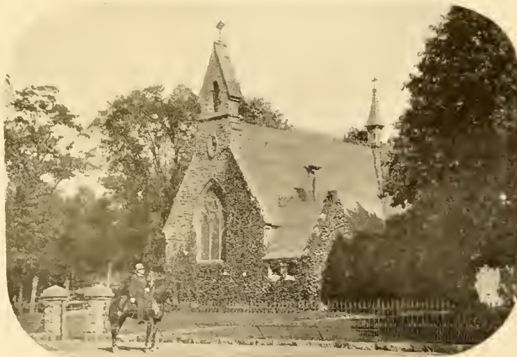
Christ Episcopal Church, Riverdale and Alamo Avenues
