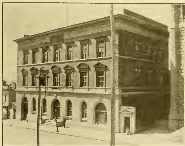
Thirty-Seventh Precinct Police Station, Bathgate Avenue near 177th Street
