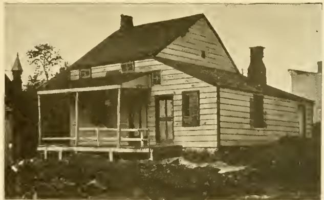
Old Williams' House, Williamsbridge
